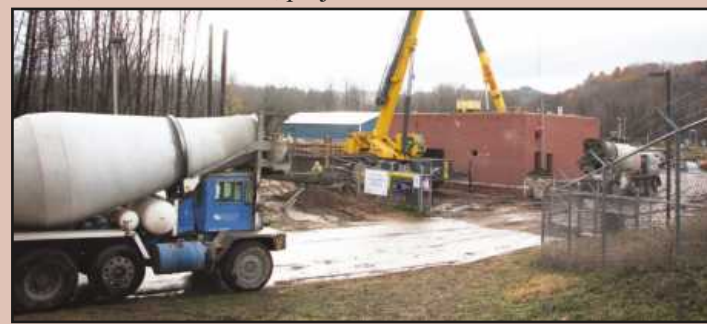
THE MARQUETTE AREA Wastewater Treatment Facility is undergoing a $14 million upgrade.
